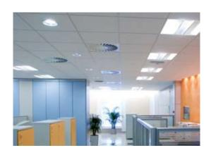
Recess mounting direct/indirect decorative mirror optics luminaire with side mirror & specially designed anodized aluminium wings suitable for 4x14W/ 4x24W FTL for modular/Armstrong/POP/Gypsum board false ceiling.
