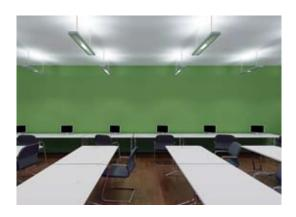
Surface mounting decorative mirror optic luminaire suitable for 2x36W (T8) linear fluorescent lamps.
