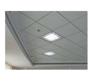
Recess mounting decorative luminaire with Paralite P5 louvre suitable for 2x36W FP-L or 3x36W FP-L designed for Modular/ Armstrong/ POP/ Gypsum board false ceiling.
