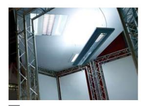
Surface mounting decorative mirror optic luminaire suitable for 1x36W (T8) linear fluorescent lamp.
